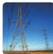
Electric Power Engineering
